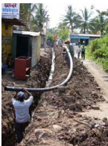
Fig. 1. Installation of PE100 pipes in progress at Malkapur
