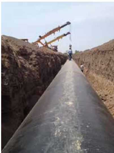
Fig. 6. Installation of 3LPE coated steel pipes in GWIL project.
