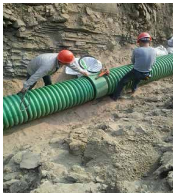
Fig. 4. Installation of PP DWC waste water pipes at the chemical park in China.
