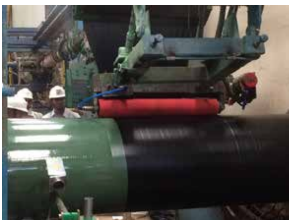
Fig. 7. 3LPE coating of steel pipes in progress.
