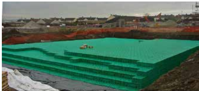
Figure 11. Installation of infiltration boxes, courtesy of Pipelife
