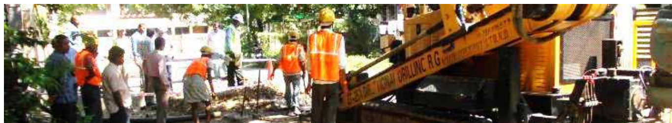
Fig. 2. Installation of PE100 pipes by HDD technique at Nagpur Veolia project
