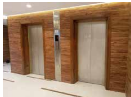
Figure 6: Wall Decorate With LVT
