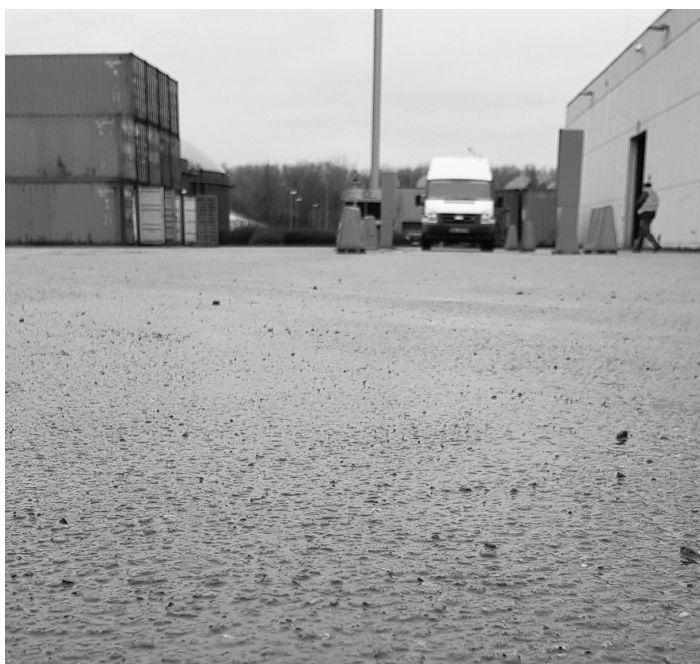
Figure 10 - Rubber-modified industrial area in Germany after 11 years of heavy traffic load
